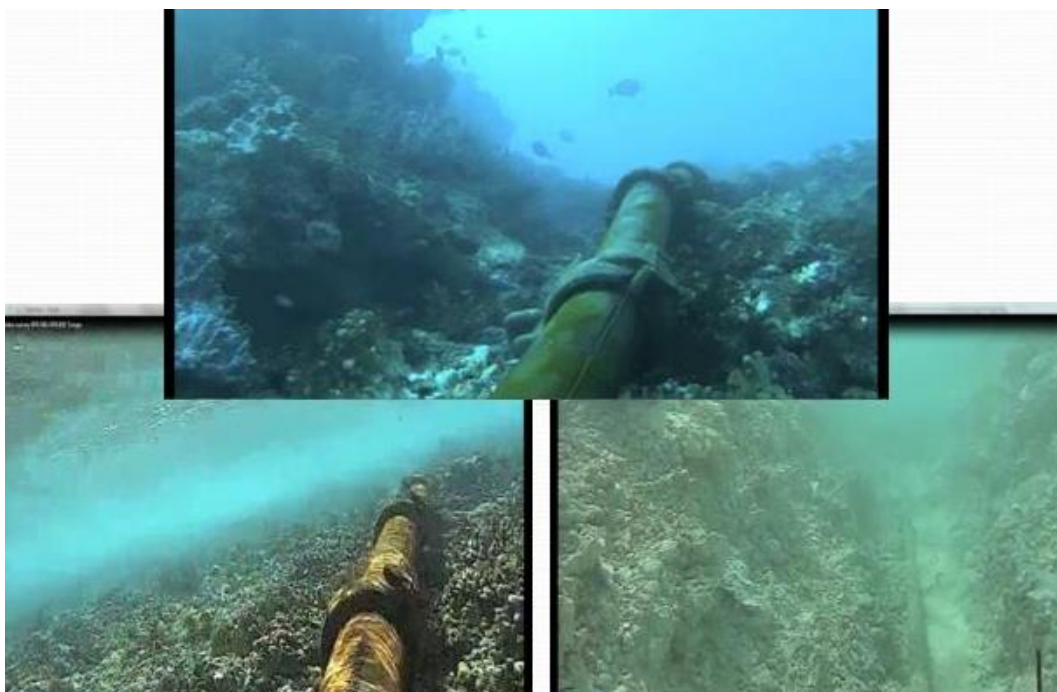
Figure 6: Tonga Cable Submarine Fibre Optic Cable Laying on Seabed 11
